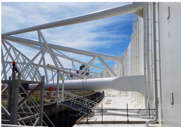
Figure 8. The Maeslantkering storm surge barrier.
